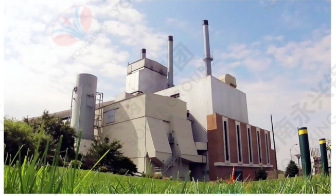
2016.02 安徽亳州广印堂中药20吨循环流化床锅炉 2016.02 20t/h CFB boiler in Bozhou Guangyintang pharmaceutical factory
