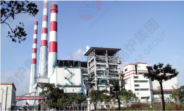
2004.11 山东日照圣运化工35吨循环流化床锅炉 2004.11 35t/h CFB boiler in Rizhao Shengyun chemical factory
